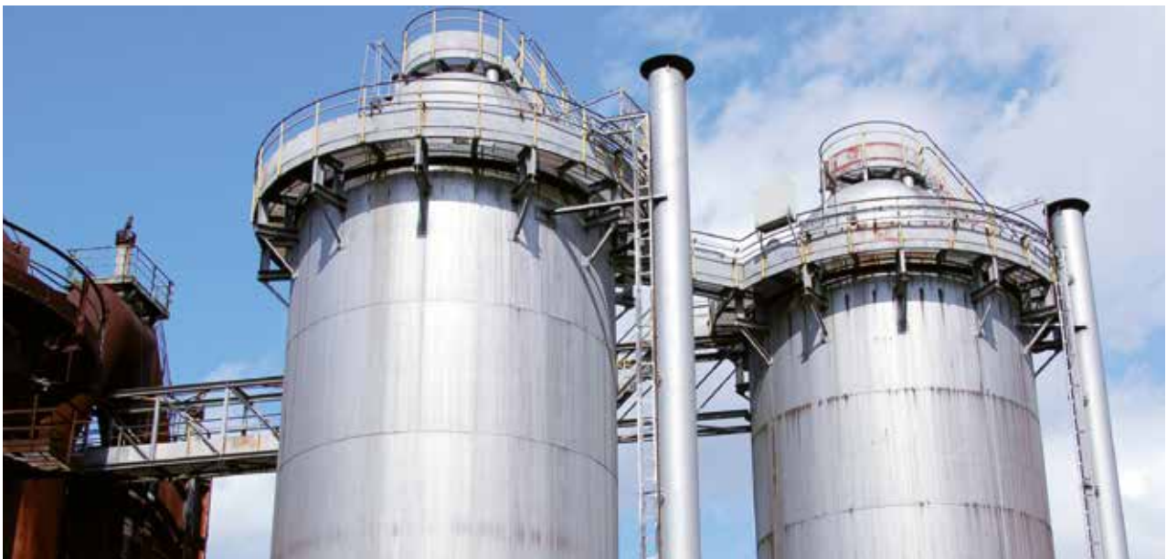
Silo loading and unloading
