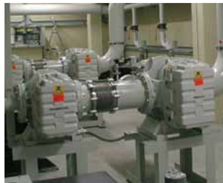
3-stage pumping set for 2 x 12,000 m 3 /h in vacuum coating technology
