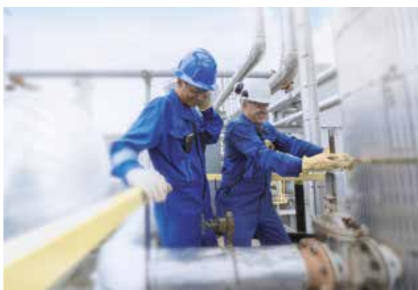
Installation at site by our technicians
