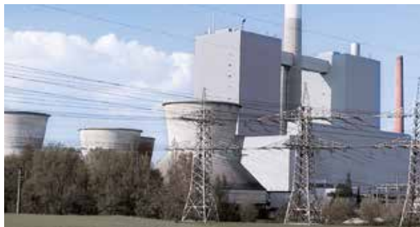
Indispensable for power plant
