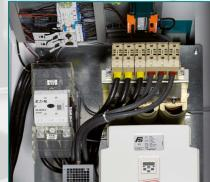
The frequency converter is integrated in the cool, dust-free area of the system.
