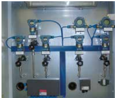
Intrinsically safe special transmitter instrumentation - for use in hazardous areas
